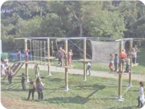
Each module measures up to 4x3x4m and the structures can be configured in different ways:
